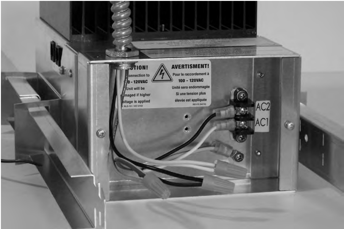
Figure 10: Completed Wiring in Junction Box
